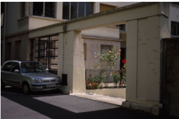
Gorska, 3, rue Casimir Pinel, Neuilly, 1931, auto ramp to underground garage.
